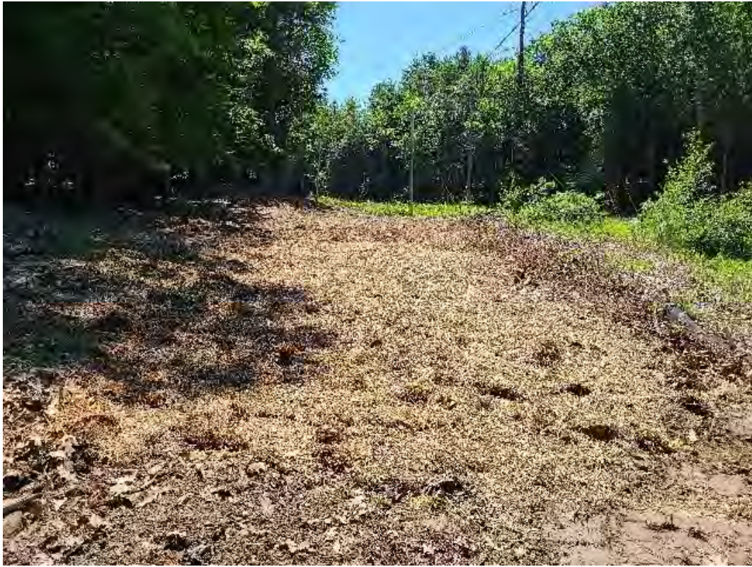
Fig 1: Removing gravel access road between Strs. 97-98. Viewing east. (07-02-20).
