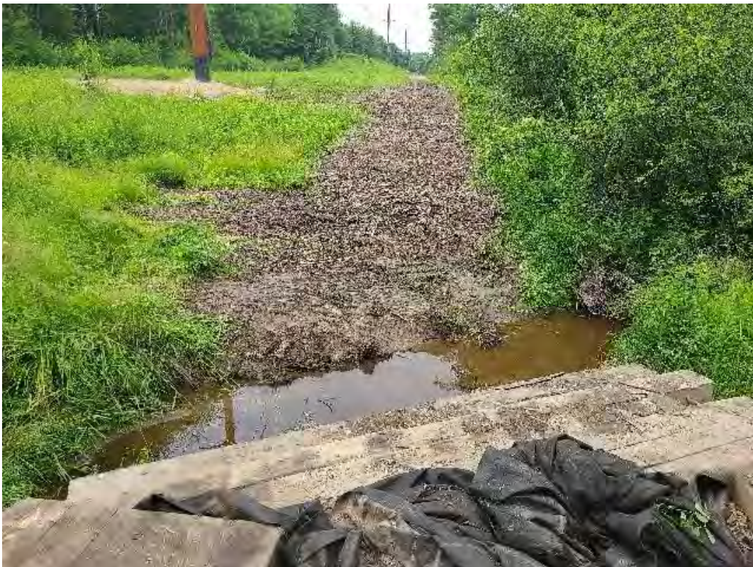
Fig 8: Removing timber mat bridge over stream DS60, between Strs. 44-45. Viewing north. (07-08-20).
