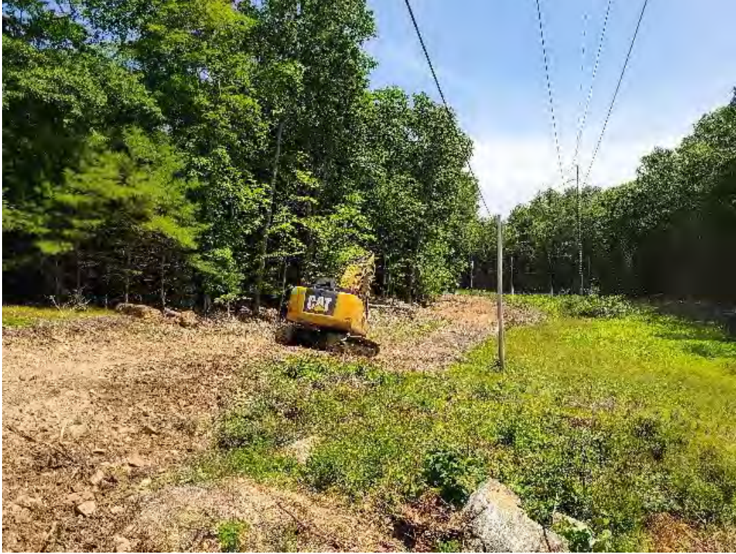
Fig 5: Crew continues to remove stone access road between Strs. 95-96. Viewing southeast. (07-07-20).
